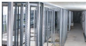
Drywall tracks to concrete and steel
