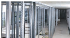
Drywall tracks to concrete and steel
