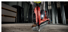
Fastening wood, e.g. Placopan®, to concrete
