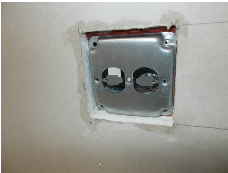
Fig. 4 Variant 4, metal box for electrical installation sealed with HILTI Putty Pad with metal cover
