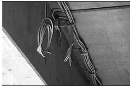
X-ECH for fastening bunched cables
