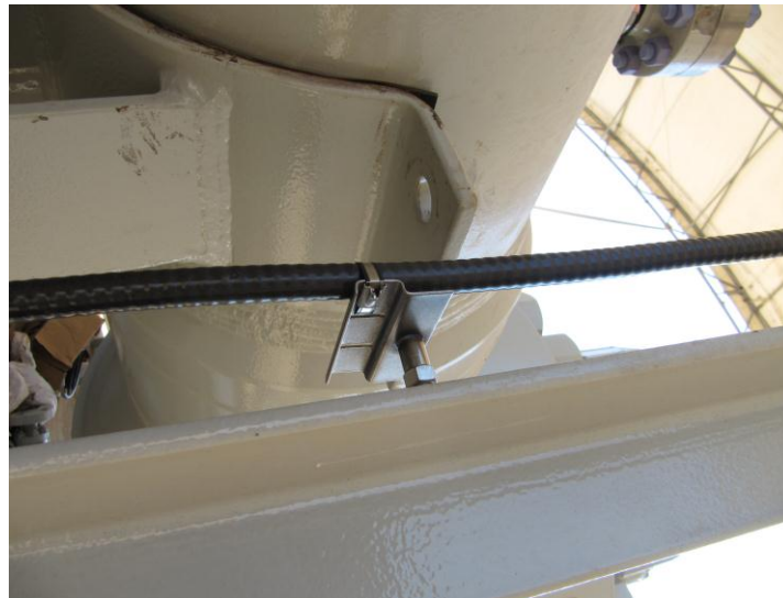
T-bar for fastening cables to steel structures
